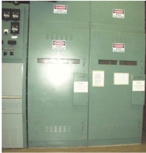
Fig. 1 WESTINGHOUSE 34.5KV LOAD INTERRUPTER SWITCH TYPE WLI
